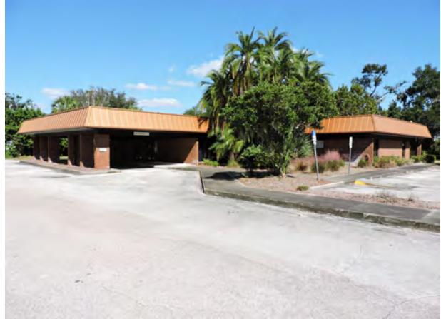
Parking Lot View
